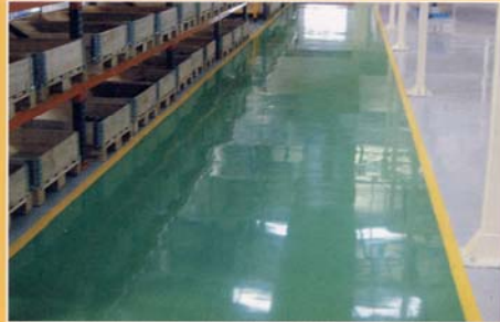
self leveling epoxy flooring
